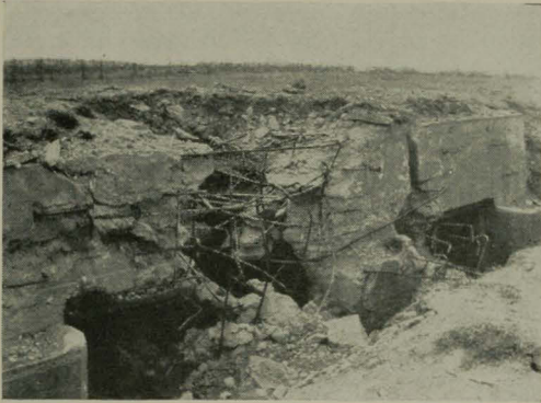
Effect of a Direct Hit on a German Concrete Shelter
